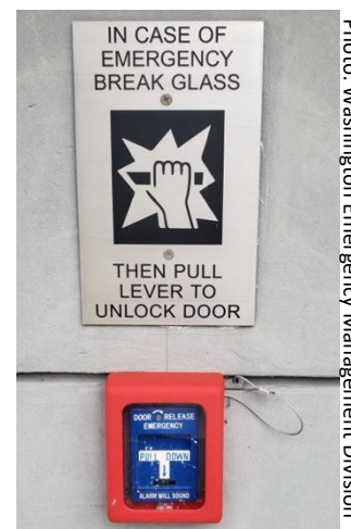
Figure 24. Emergency door release device.
